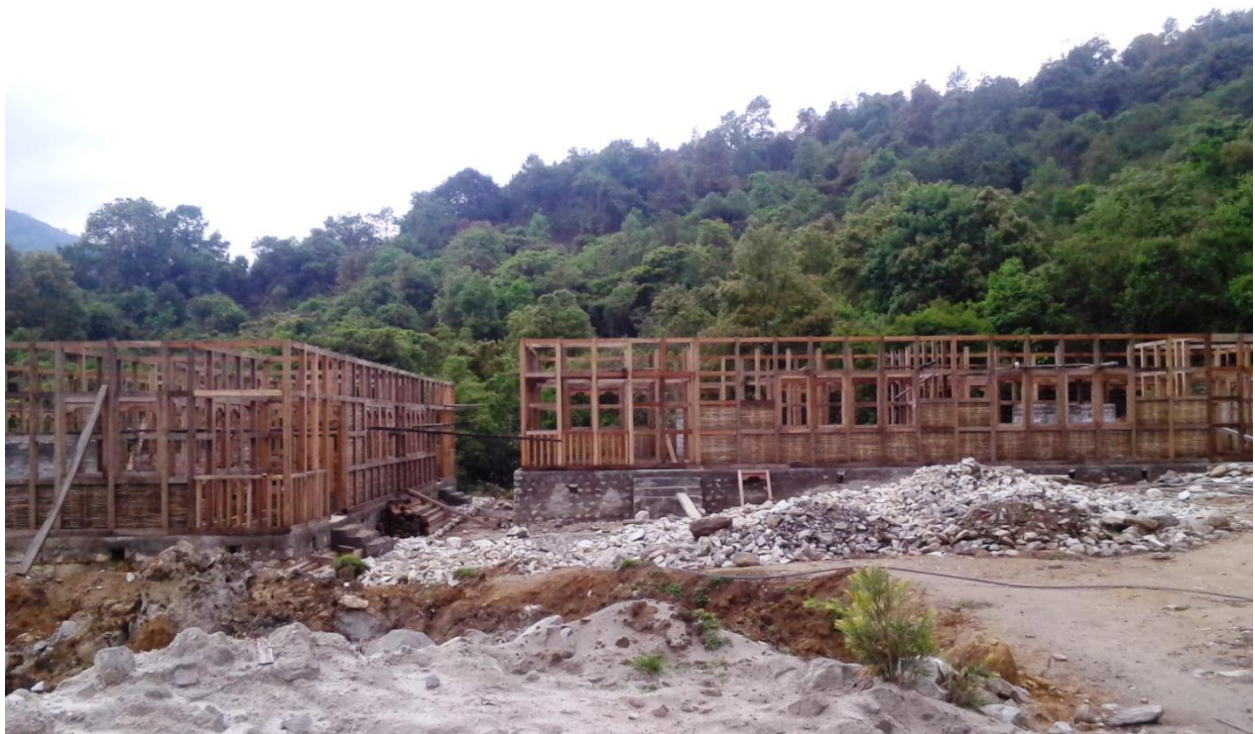
Infrastructure building in progress
