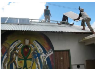
Technicians installing panels
