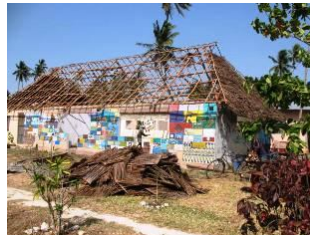
The roof half finished
